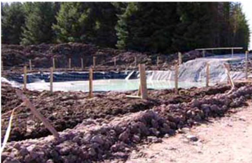
Figure 4.8: Typical Lined Settlement Pond for Concrete Wash out Facility
