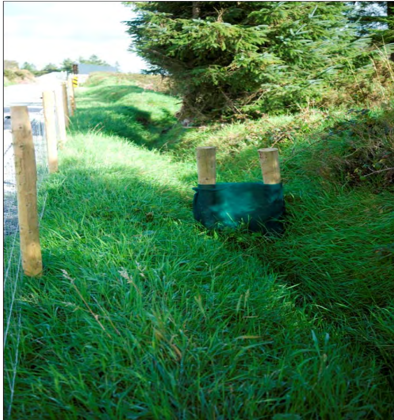
Figure 4.4: Typical Silt Trap across Grassed Swale
