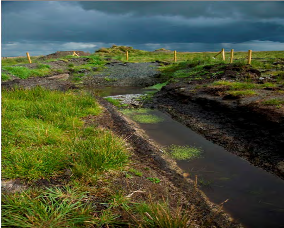
Figure 4.2: Typical Swale draining to Stilling pond
