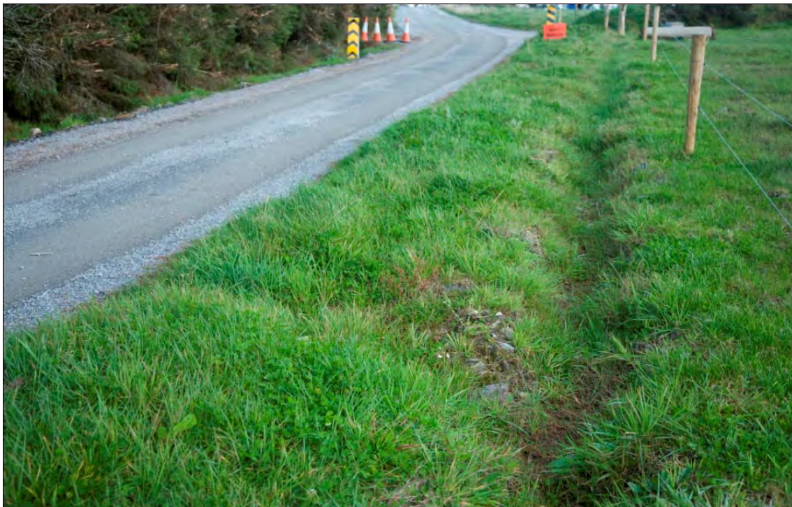
Figure 4.1: Typical Grassed Swale along access road
