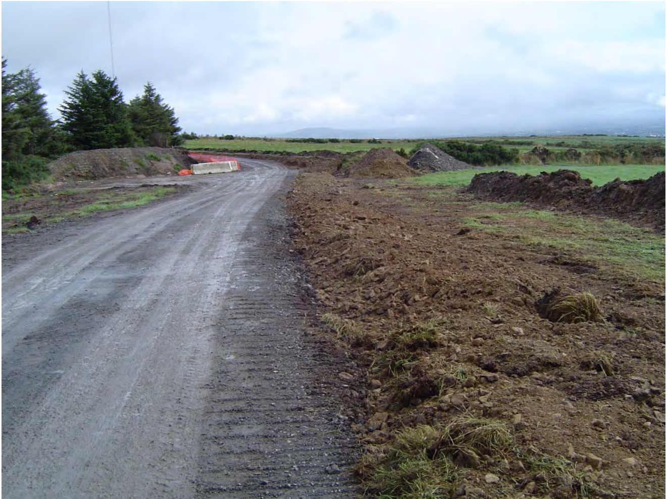
Figure 4.7: Typical Backfill Over Cable Trench
